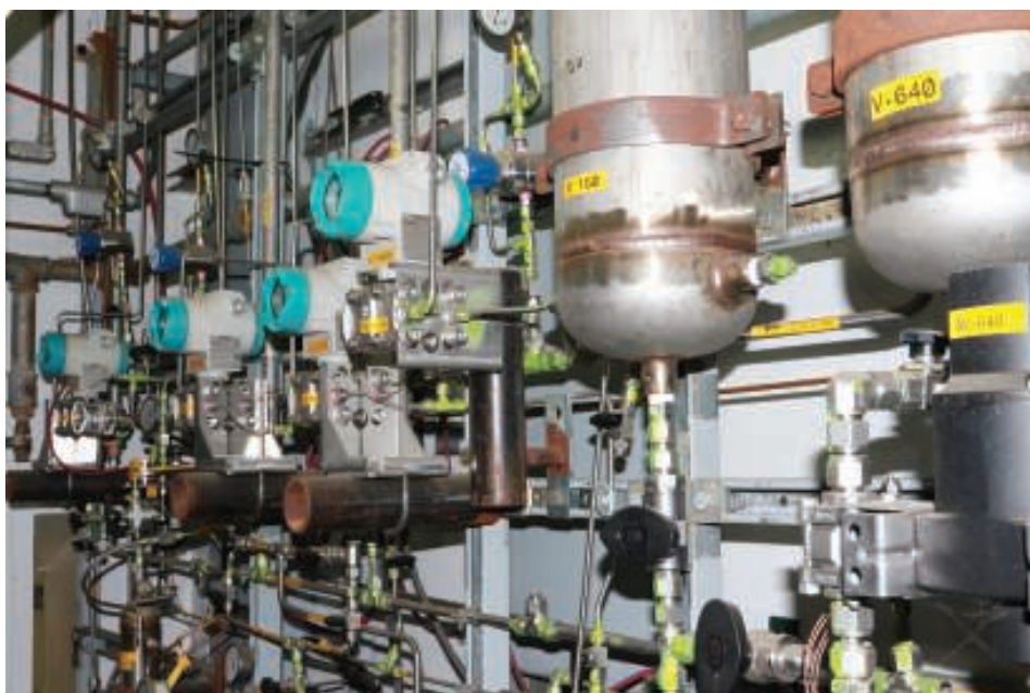
FIGURE 1. Instrumentation is one area in pilot plants that typically does not scale up — very small tanks likely still have instrumentation requirements similar to 15,000-gal tanks in a commercial plant
