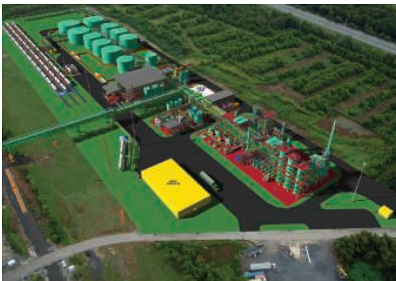
FIGURE 4. This site layout model, produced using CADWorx from Intergraph, shows piped, road and rail links
