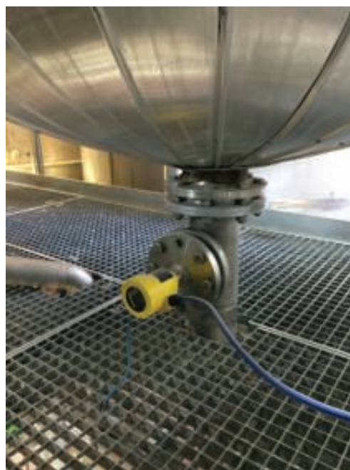
FIGURE 3. Shown here is a master sensor for an electronic DP measurement in a distillation tower
